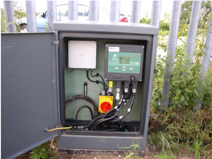
Photo 5: Control unit located in “Lucy” enclosure, no heating/cooling systems are required.
